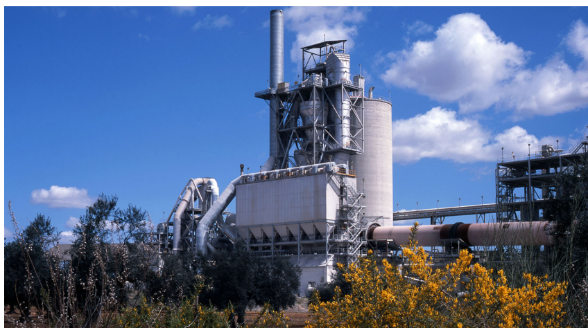
Cement factory in El Alto, in Morata de Tajuña (Madrid).
