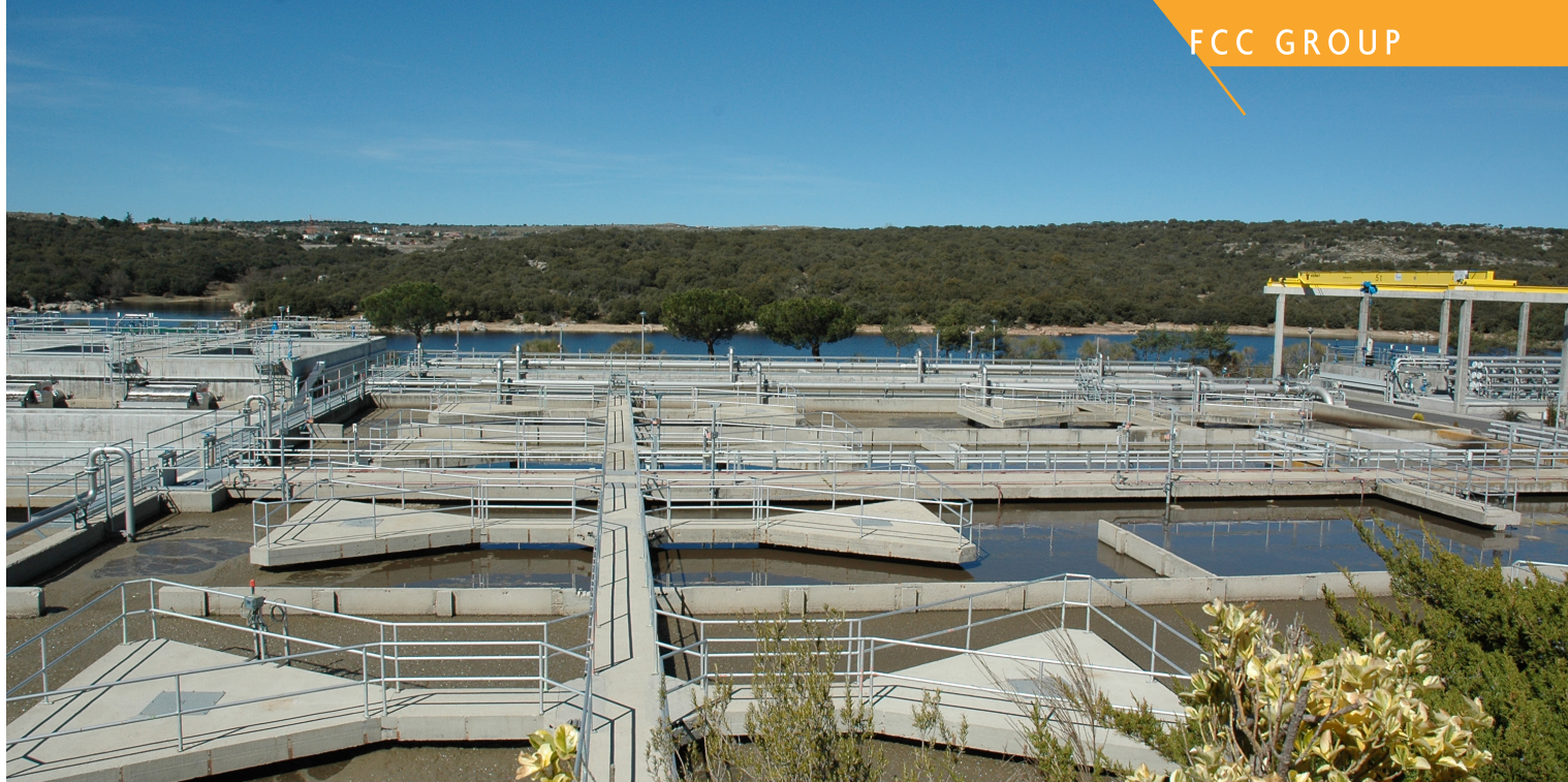
The Ávila wastewater treatment plant.
